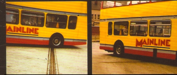
Rotherham Bus Station LR55 installation – 2400 buses a day
